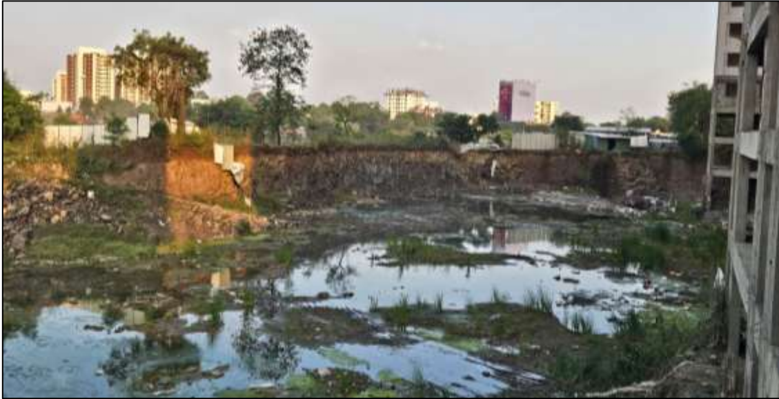
Excavation for Wing D & E is Completed
