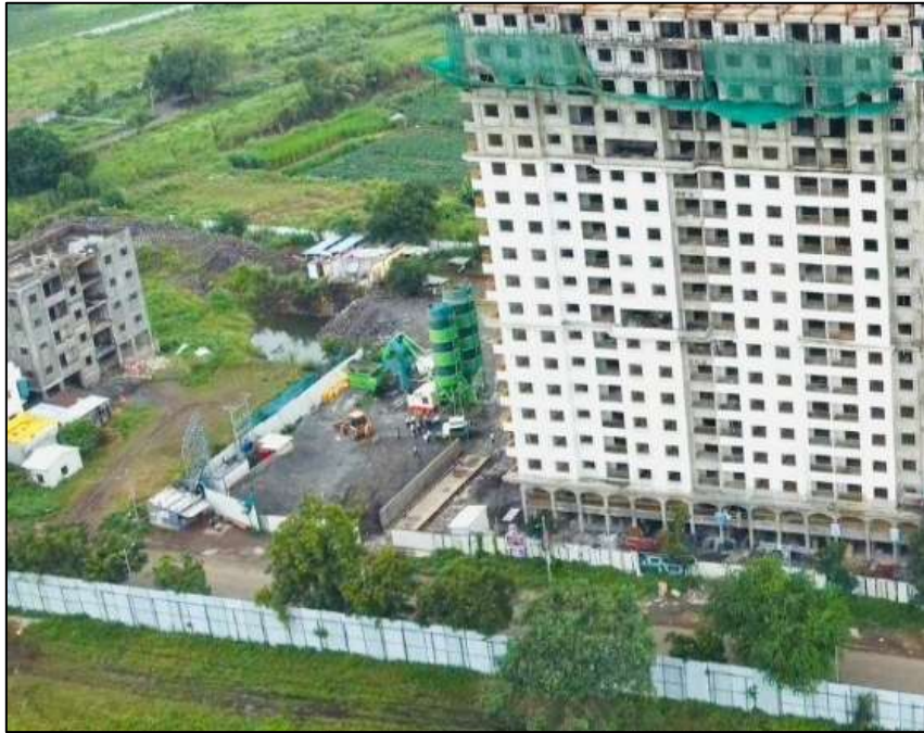
RCC of Wing B completed up to 18 th Floor,
