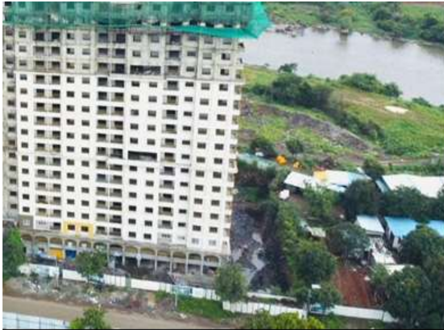
RCC of Wing B completed up to 18 th Floor,
